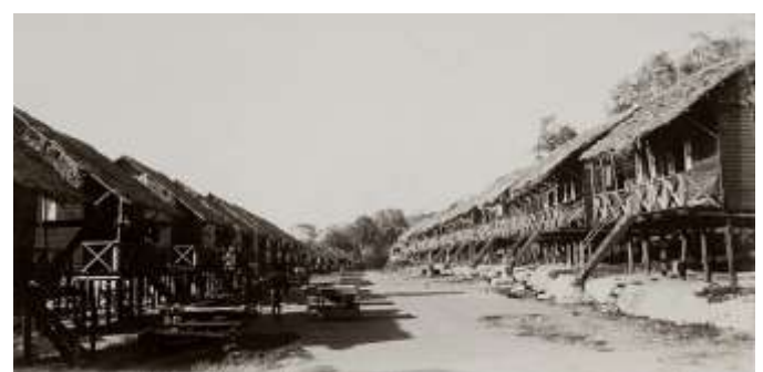
Figure 35. Left: Part of c1903 map showing coolie lines in Settlement. The "Eating Shed" for the coolies was located in what is now the parking lot across the road from the supermarket. Right: "New" coolie lines in 1905 (Extending from supermarket to Tai Pak Kong Temple, Gaze Rd) Source: https://christmasislandarchives.com/coolie-houses/ , Accessed: May 3, 2026.
