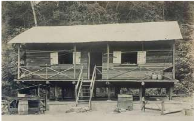
Figure 36. Photograph of most recent type of Coolie House as erected at Christmas Island. This may be taken as almost a model for this type of building (1911)
