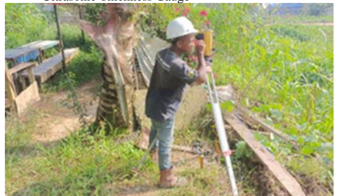
Fig. 4. Bridge situation and geometry measurement using total station.
