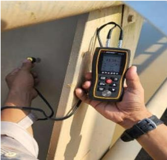
Fig. 6. Measurement of steel profile using ultrasonic thickness gauge.
