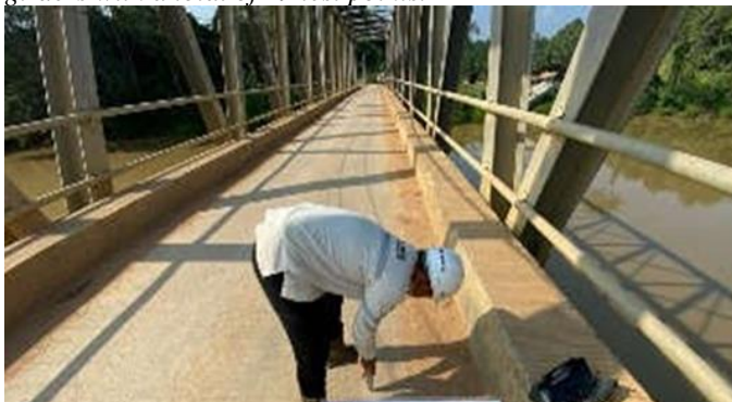
Fig. 3. Hammer test execution on bridge floor slab.
