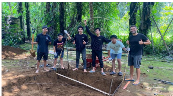
Fig.4. Mockup construction process
