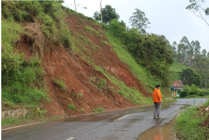
Fig. 7. The location of the landslide in the Pangalengan area is in the form of tuff rock with a slope of 35% (Sulastri, 2021)
