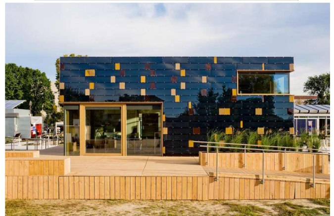
Figure 23. 2015 PROTOTYPE HOME: Technische Universitat Darmstadt team building (2009)
