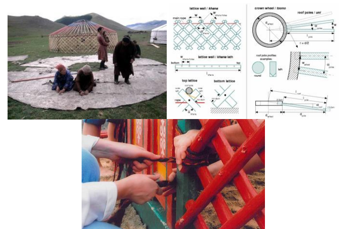
Figure 10. Yurt. Assembly of elements
