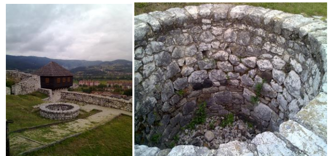
Figure 18. Water cistern (catrnja) in Doboj fortress
