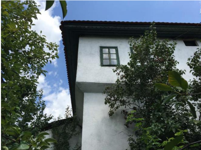
Figure 5. The Gradascevic family house in Gradacac. The impressive, huge volume of the floor, which is cantilevered into the space over the contour of the ground floor, is reminiscent of the 'white tower of Hussein-kapetan'. Source: Author (July 20, 2016)
