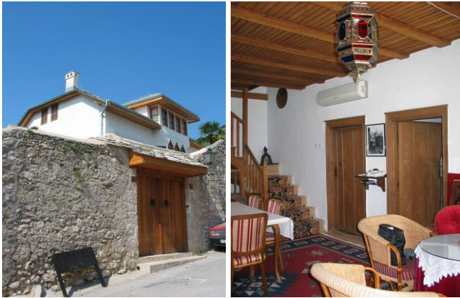
Figure 11. The Muslibegovic family house in Mostar. Left: Access gate to the inner courtyard from Osmana Đikić Street. Right: Inner door, wooden ceiling ('shishe')
