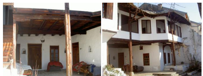
Figure 5. The Kajtaz family house in Mostar. Porches on the ground floor and divanhanes on the first floor Source: Haris Bradic (January 10, 2007)
