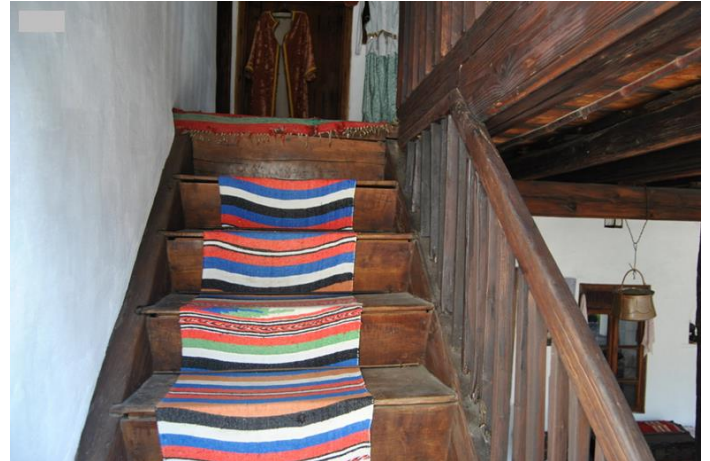
Figure 8. The Kajtaz family house in Mostar. A wooden staircase ('basamaci') connects the ground floor level with the first floor level
