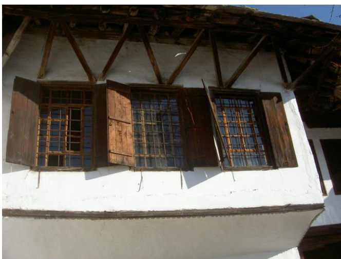
Figure 7. The Kajtaz family house in Mostar. The cantilevered projection of the volume ('doxat') outside the contour of the ground floor
