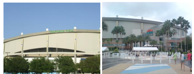
Figure 10. 'Tropicana Field (Suncoast Dome)', Saint Petersburg, Pinellas County, Florida (1989), (Architects: HOK Sports Facilities Group, Constructors: Geiger/KKBNA)
