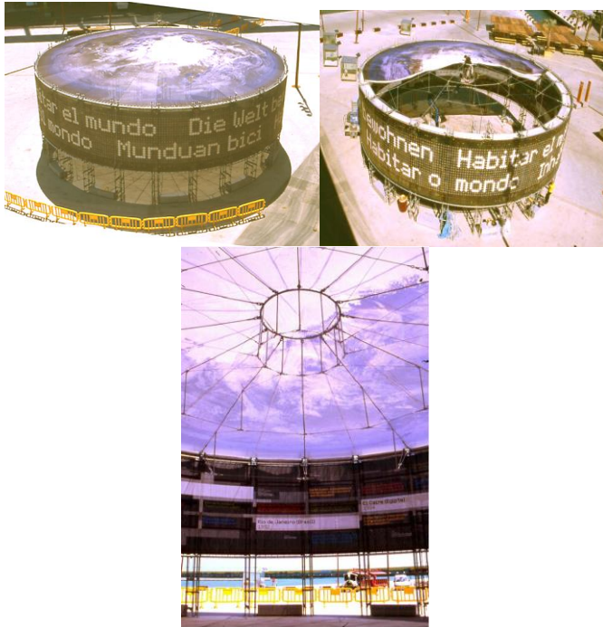
Figure 13. 'Bifid Tension Dome', Marina Seca, Barcelona, 2004 (Architects: Guri & Casajuana, Constructors ARQINTEGRAL (Ch.García-Diego & H.Pöppinghaus) with J.Llorens)
