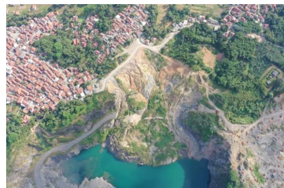
Fig. 6. Aerial Photographs Using Drones in Landslide Areas
