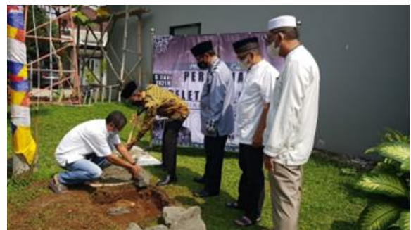
Fig. 2. Renovation and laying of stones at the At Taqwa Erfina Kencana Regency Mosque In 2021 by the Chairman of the DPRD Kab. Bogor
