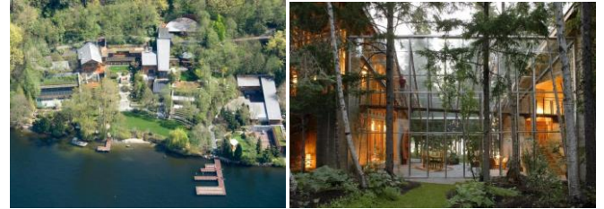
Figure 27. Bill Gates house, Medina, Lake Washington, Seattle, USA (1992-1994. Architects: James Cutler and the architectural firm Bohlin Cywinski Jackson)
