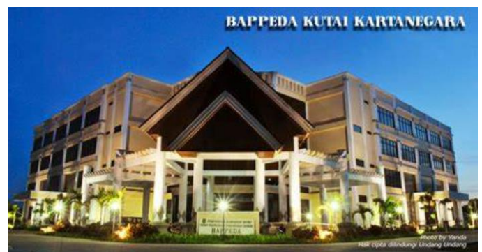
Fig. 2. The front view of the building
