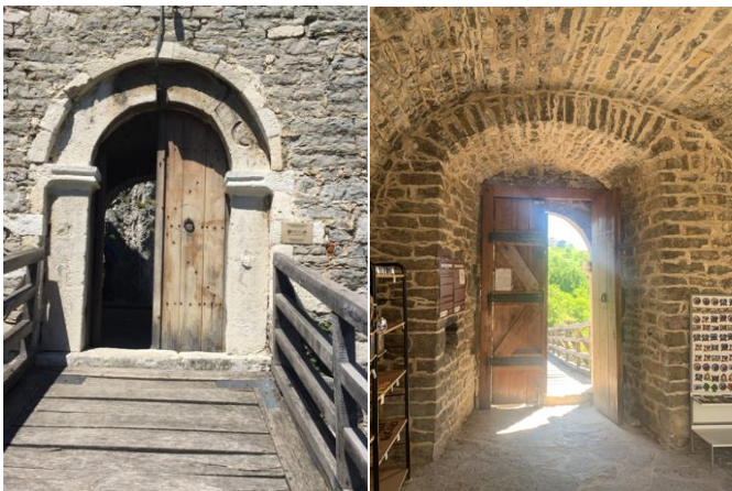
Figure 5. Entrance to the Old Town Srebrenik. View of the entrance from the access bridge (left) and view from the entrance tower towards the access bridge (right)
