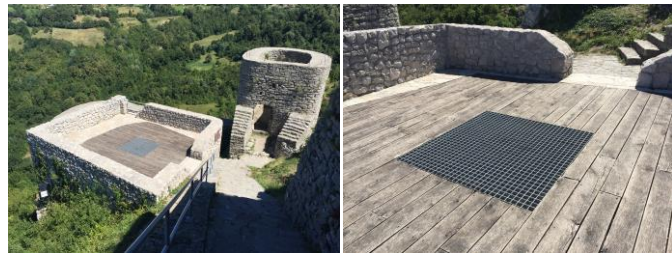
Figure 8. North tower (remains of the former mosque)
