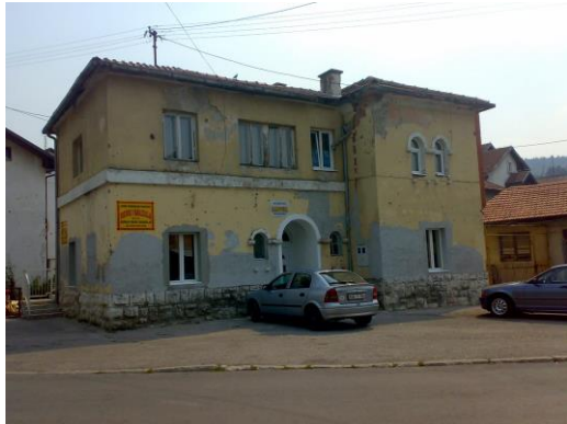
Figure 16. Administrative building of the Public Utility Company Sana Source: http://mojpokusaj.blogspot.com/2012/08/ , Accessed: 8.6.2022.
