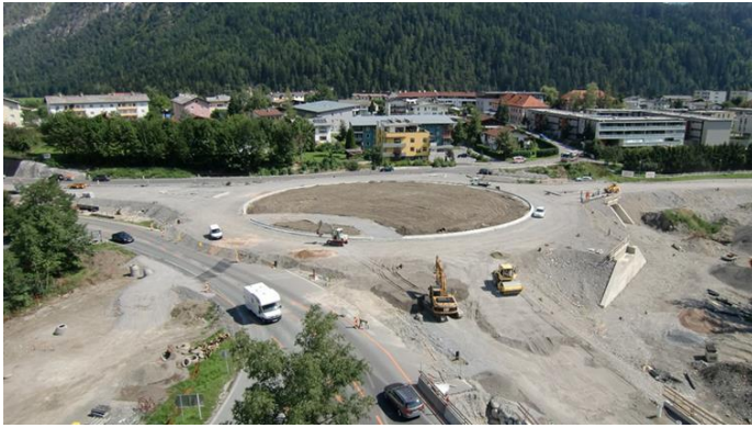
Figure 2. Aerial view of the Imst roundabout on Arzil during construction [5]
