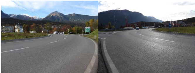
Figure 6. View towards the entrance and exit of the B189 Reutte/Garmisch (GER) [6]
