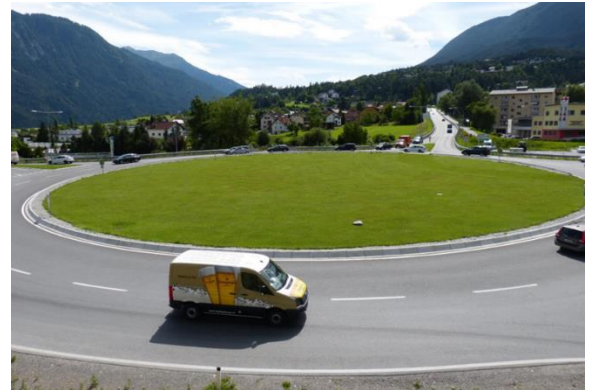
Figure 3. Finished roundabout Imst on Arzil [5]
