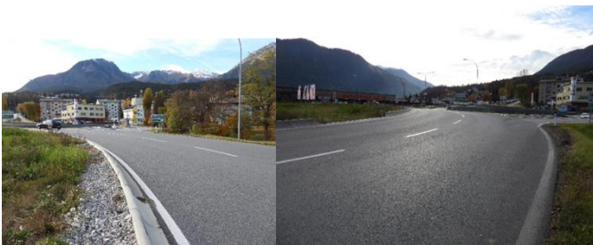
Figure 8. View towards the Hoch/Imst-Centre entrance and exit [6]
