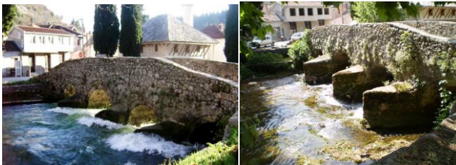
Figure 18. The Spite Bridge ('Inat Cuprija') in Stolac (17th century) Source: https://www.tourguidestolac.com/inat-cuprija/ , Accessed: 7.30.2022.
