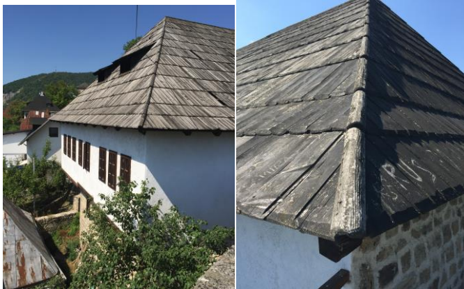
Figure 13. Krslak's house 01. Left: vertical composition of the house. Right: roof
