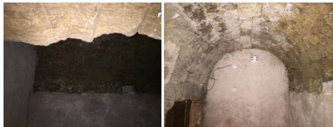
Figure 15. Krslak's house 01. The warehouse in the basement is mostly carved into the rock
