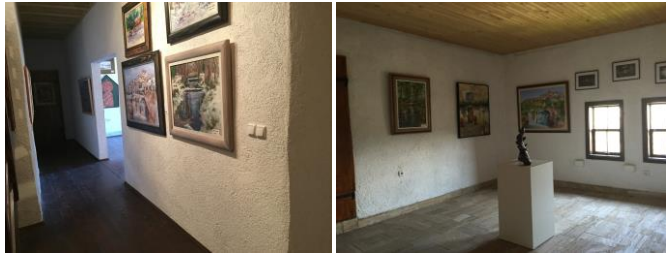
Figure 24. Krslak's house 01. Today's condition and purpose of the building. City Gallery
