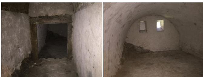
Figure 9. Krslak's house 01. Left: access to the ground floor space 'built' into the rock on the spot. Right: 'carved' space in the rock in situ (ground floor level)
