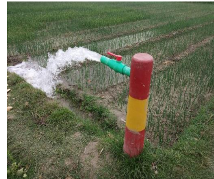
Fig. 3: Supply of irrigation water through dug well's faucet connected with underground uPVC pipe line.
