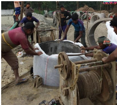
Fig. 1: Lowering of dug well ring.
