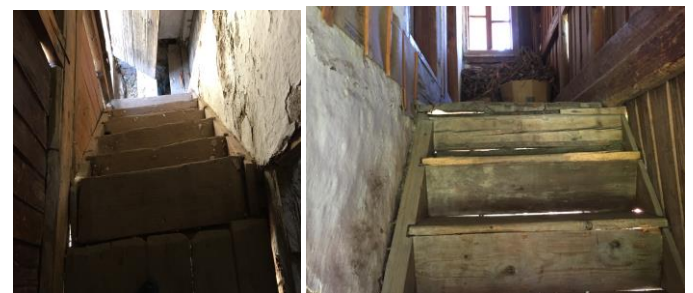
Figure 19. The Colak family house in the Brnjic village near Kakanj. Wooden one-legged staircase ('basamaci') Source: Author (June 28.2016.)
