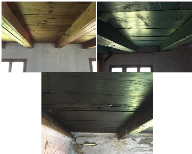
Figure 21. The Colak family house in the Brnjic village near Kakanj. Left and center: floor-attic construction. Right: ground-floor (hewn beams and wooden floors)
