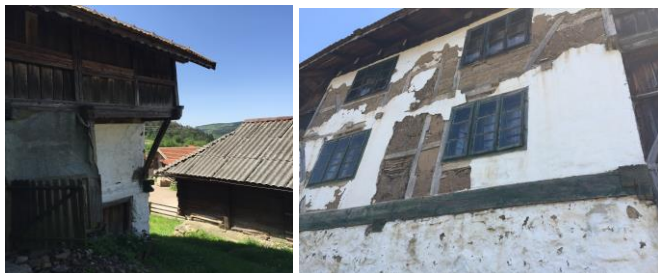
Figure 10. The Sljivo family house in the Brnjic village near Kakanj. Structure of the house: stone wall of the basement, wooden skeleton with adobe filling on the ground floor and first floor Source: Author (June 28.2016.)
