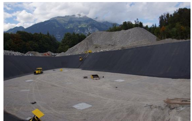
Fig. 16. Asphalt work at the Cholwald landfill site [2]
