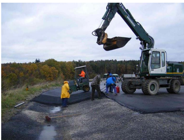
Fig. 24. Asphalt trough installation of the Ramsklunge landfill site [21]
