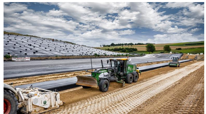
Fig. 21. Paving and compaction at the landfill "Abfallentsorgung Kreis Kassel", Germany [19]
