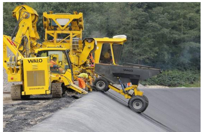
Fig. 15. Asphalt work at the Cholwald landfill site [2]
