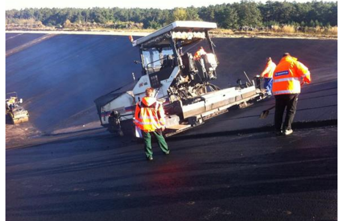
Fig. 32. Installation of DAD in the embankment area [22]
