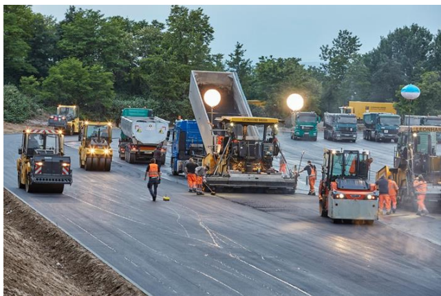
Fig. 18. Asphalt paving at Vogelsang landfill, Heilbronn, Germany [17]
