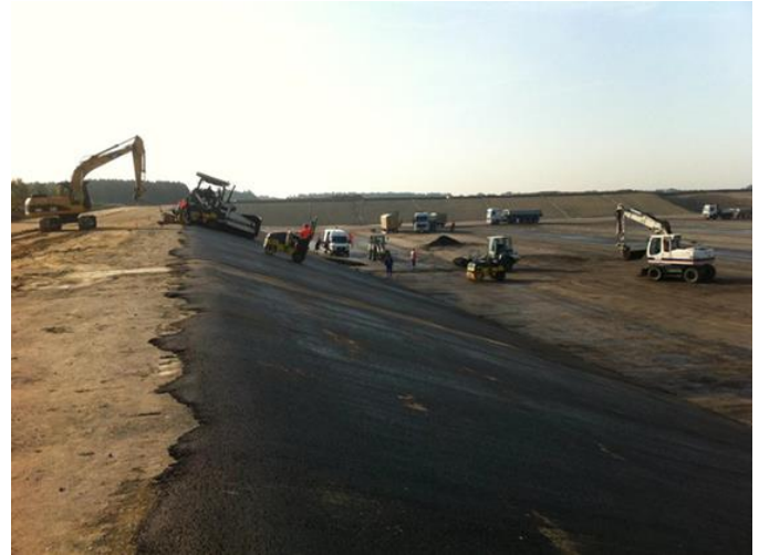
Fig. 30. Installation DAT in the slope area [22]
