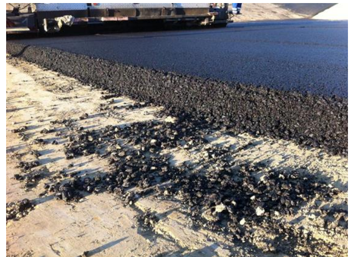
Fig. 31. Installation DAT in the embankment area, detail [22]
