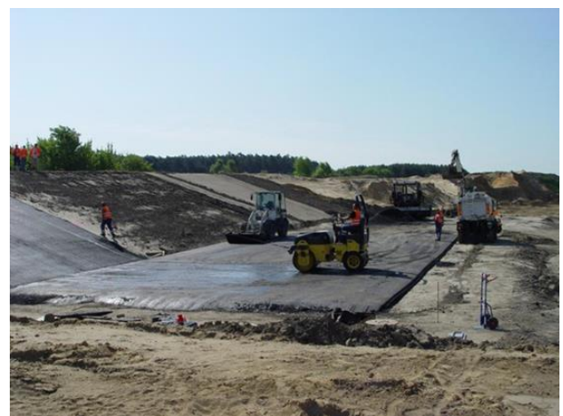
Fig. 26. Construction 1st test field [22]
