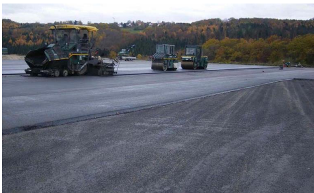
Fig. 23. DAD – installation in the leveling area of the Ramsklunge landfill site [21]
