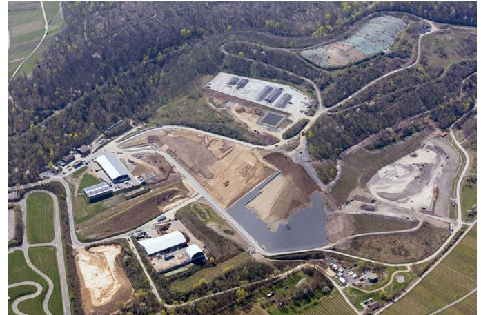
Fig. 20. Aerial view of Vogelsang landfill, Heilbronn, Germany [18]
