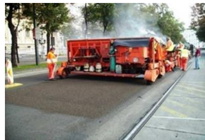
Figure 8a. Machine spreading of the hard chippings [1]
