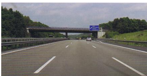
Figure 10 b) One year after installation, the brightening is clearly visible, as here on the A 61 at the Wehr exit. [7]
