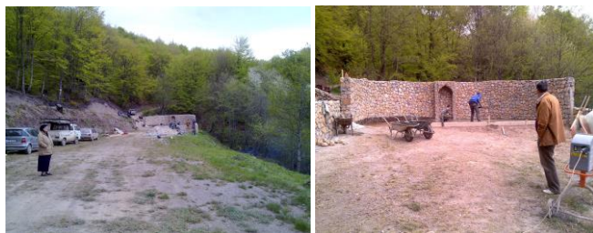
Figure 14. Musalla "Dobre Vode" (Contractor and foundation Fadil Budnjo, B.Sc. Eng. Geol.)
