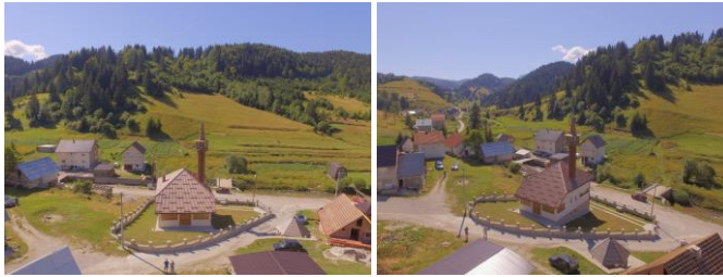
Left: Drone-camera view from the northwest direction Right: Drone camera view from the west
