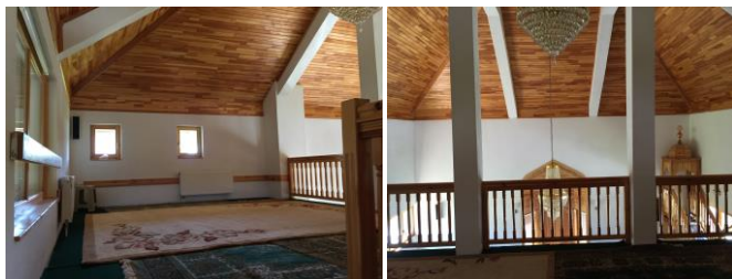
Left: View of the mahfil from the staircase Right: View from the mahfil to the mihrab and member
