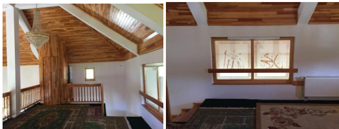
Left: View from the mahfil of the staircase and access to the minaret Right: View from the mahfil towards the window facing the entrance hall
