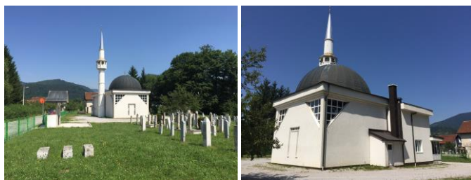
Left: View from the southeast Right: View from the southwest direction. The design of the mosque Figure 4. Mosque in Japalaci near Tarcin (1989-2007) Source: Author (July 14, 2017)
