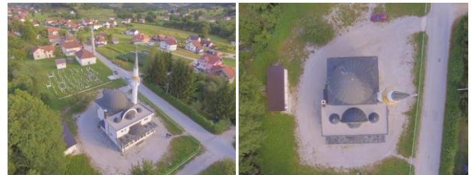
Left: Drone camera view from the north Right: Aerial view with a drone camera (Fifth facade) Figure 5. Mosque in Japalaci near Tarcin. Take photos with a drone camera Source: Vladimir Obradovic (July 27, 2017)
