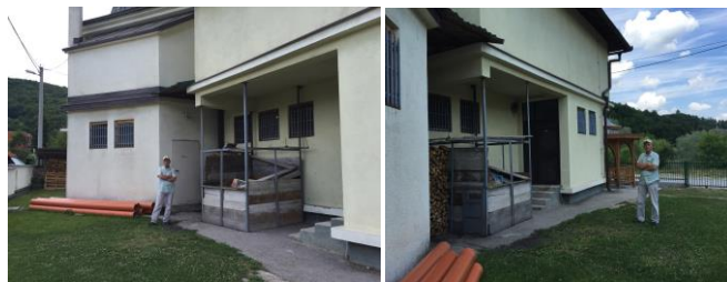
Left: Economic part of the harem of the mosque. Boiler room for central heating
