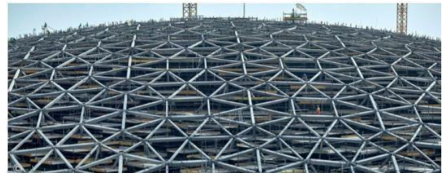
Fig. 20. Roof structure of Louvre (Moly, 2019)
