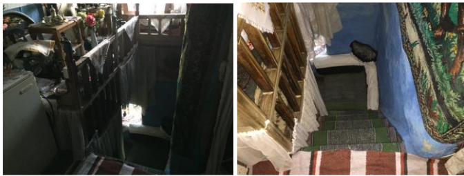
Figure 5. Wooden staircase (basamaci) and divanhana facing the street Source: Author (7.9.2016.)
