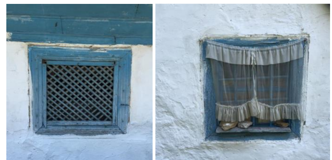
Figure 9. Windows on the ground floor
