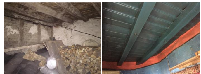
Left: Construction ground-floor (visible from the woodshed on the ground floor)
