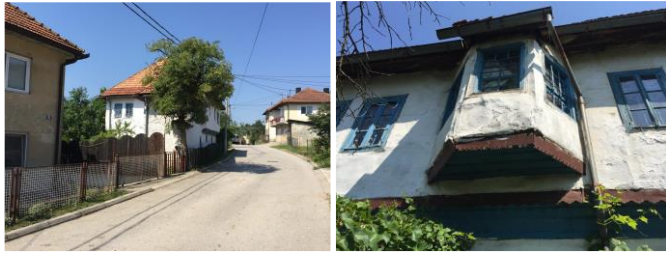
Left: View of the house from the northeast Right: Doksat divanhana facing the garden
