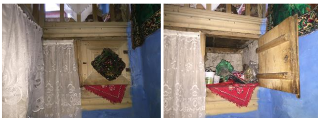
Figure 19. Niche in the wall (“dulaf”) in the area of the staircase and divanhana facing the street Source: Author (7.9.2016.)
