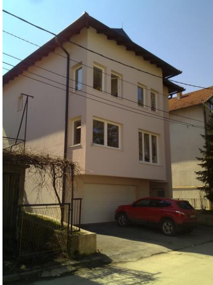
Figure 25. The A&E Hujic house, Sarajevo (2008). Photographs
