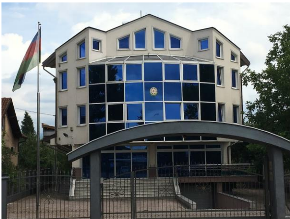
Figure 3. The M. Ahmetpahić villa (today it is the Embassy of the Republic of Azerbaijan), Ilidza near Sarajevo (2008). Photos Source: https://lh5.googleusercontent.com/p/AF1QipMb-1Ch80jDNfatiLcIE-SVT31yqyQ_xZ3ti2_e=h720 , Accessed: 3.19.2019.
