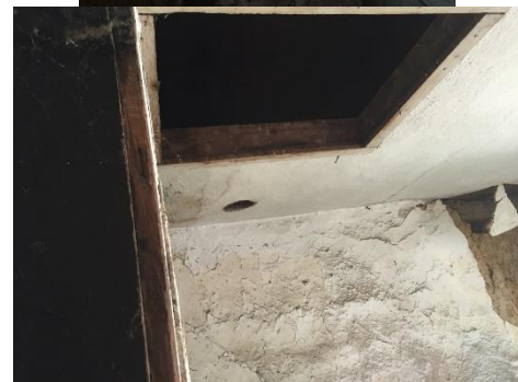
Figure 19. Hallway of the residential floor on the first floor (left) and exit to the attic space, in the hallway on the first floor (right) Source: Author (7/22/2016)
