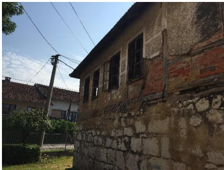
Figure 20. Construction and materialization of walls
