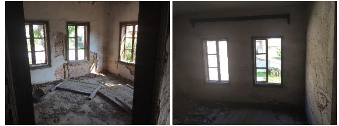
Figure 17. Chardak with street view (left) and chardak with garden view (right)
