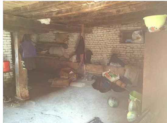
Figure 9. Former proctor barn (ground floor), now large pantry
