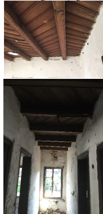
Figure 23. Wooden ceiling (bottle) in one of the balconies (left) and in the hallway of the floor (right)
