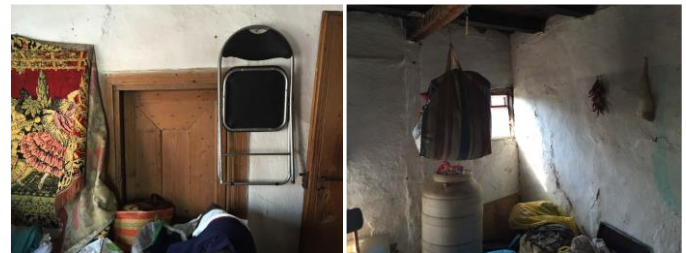
Figure 10. Hamamjik door in one of the balconies (left) and demolished space of one of the hamamjiks (right), now a pantry
