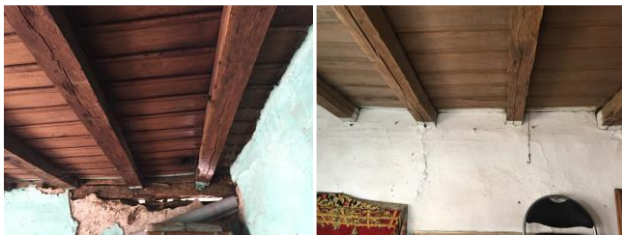
Figure 8. Floor-attic construction in the chardaks area
