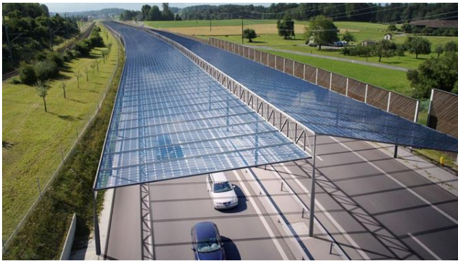
Fig. 4. This is what a photovoltaic roof for highways should look like one day [5]
