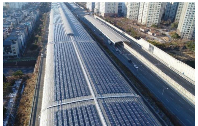
Fig. 2. Views of the soundproof housing in Korea with attached PV modules [2]
