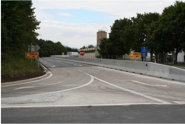
Fig. 15. Highly stressed traffic areas with semi-rigid pavement [7]
