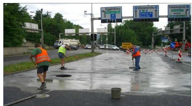
Fig. 14. Highly stressed traffic areas with semi-rigid pavement [7]
