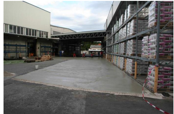
Fig. 11. Industrial bearings with semi-rigid pavement [7]
