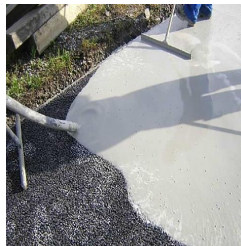
Fig. 7. Completely penetrated with the mortar [7]
