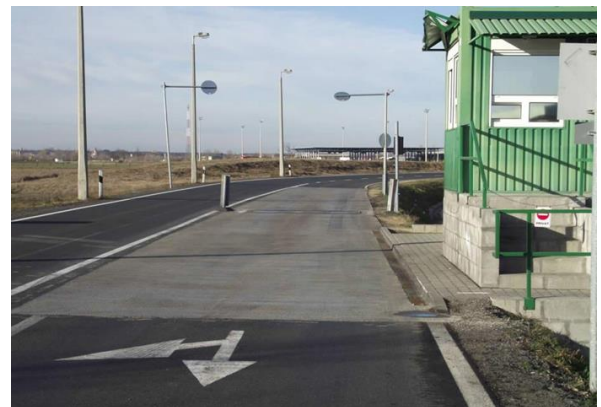
Fig. 13. Highly stressed traffic areas with semi-rigid pavement [7]
