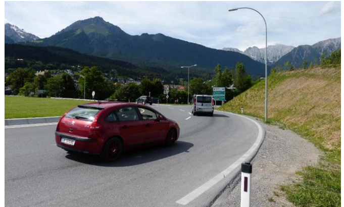
Fig. 2. Bending in the circular roadway [4]
