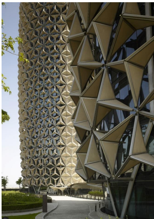
Fig. 7. Al-Bahr Tower, shading devices [30]
