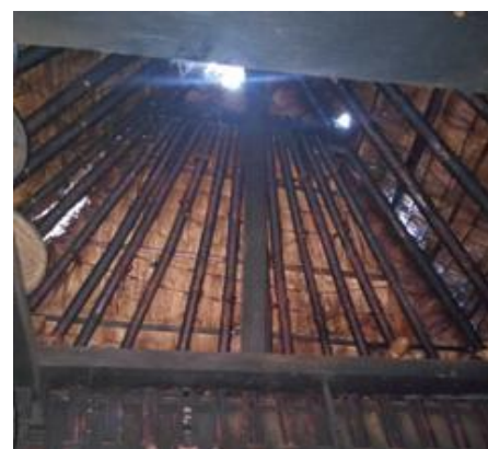
Fig. 8. Structure of Bale Bayan's roof
